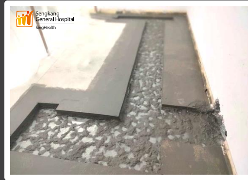
Waterproofing and lead-lining works of the walls and floor
